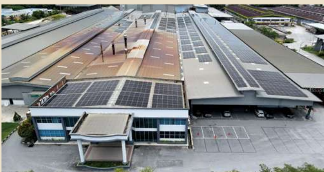
Figure 1: Rooftop solar PV system at Plant 1
