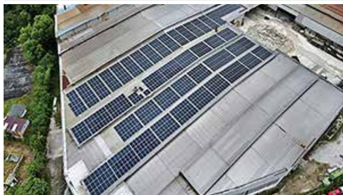
Figure 3: Rooftop solar PV installed at KHCS Plant 2
