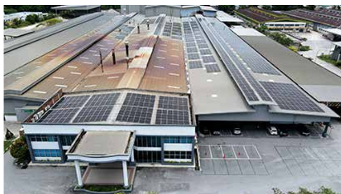
Figure 1: Rooftop solar PV system at Plant 1
