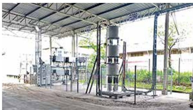
Figure 2: Metering and Breaker Panel, Inverter Station and Fault Current Limiting Reactor (FCLR) at KHCS Plant 1
