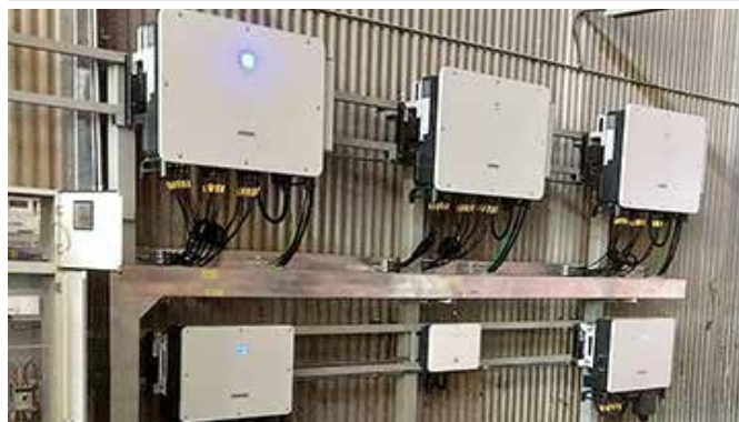
Figure 4 : Metering and Breaker Panel and Inverter Station at Plant 2
