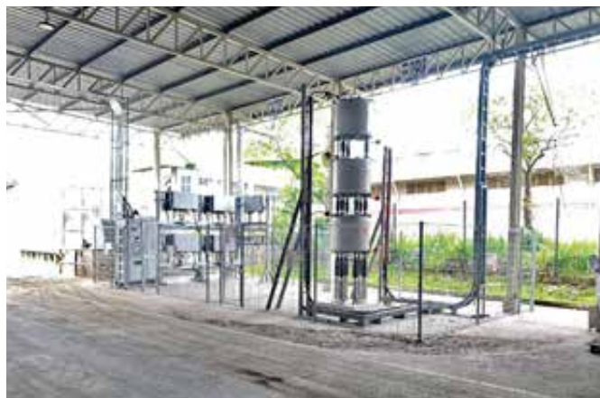
Figure 2: Meter and Breaker Panel, Inverter Station and Fault Current Limiting Reactor (FCLR) at KHCS Plant 1
