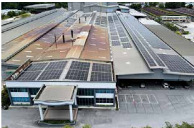
Figure 1: Rooftop solar PV system at Plant 1
